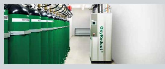
also able to maintain the reduced oxygen concentration for as long as is desired after quick release has already been carried out. WAGNER and VdS have conducted special joint fire tests with the quick release unit to document the system's reliability. This led VdS to test the system installed in the Lenbachhaus and approve it.
