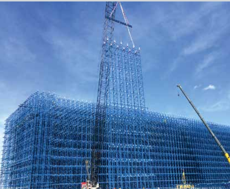
The logistically efficient, clad-rack structures are not yet as common in the US as they are in Europe.
