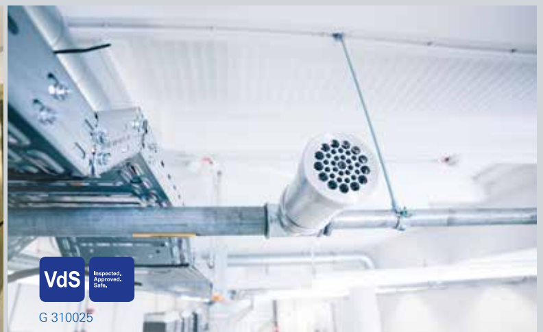
Special sound absorbers are attached to the extinguishing nozzles
